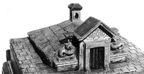
Well chamber of Hernalds water pipeline
