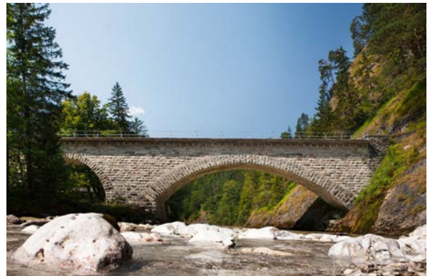
Aqueduct of 2 nd Spring Water Main across Salza river
